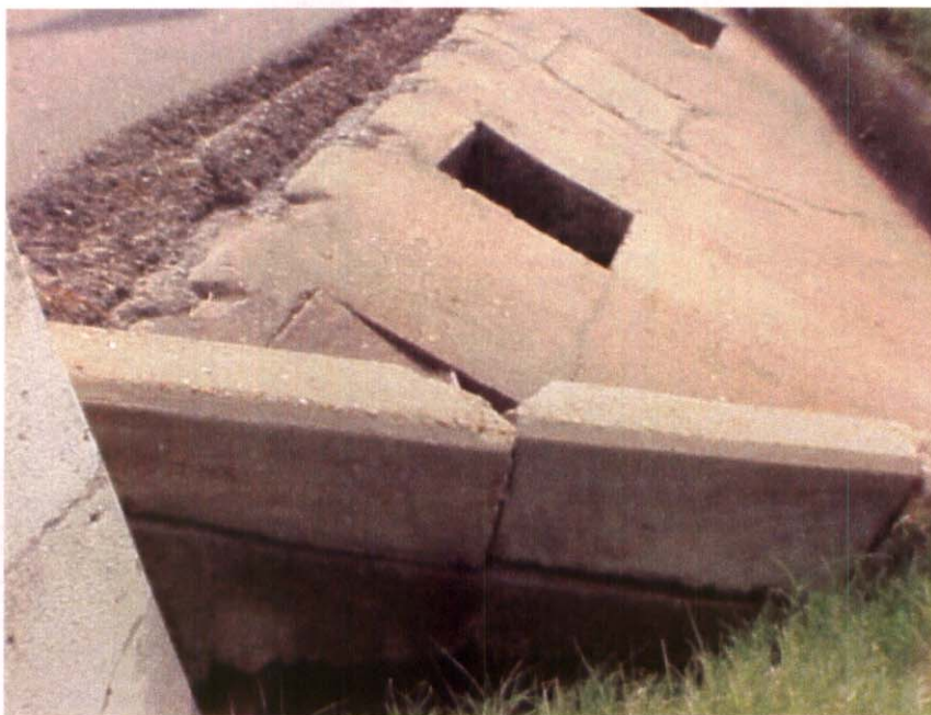
APPROACH #2 EMBANKMENT WASHING UNDER DRAIN
