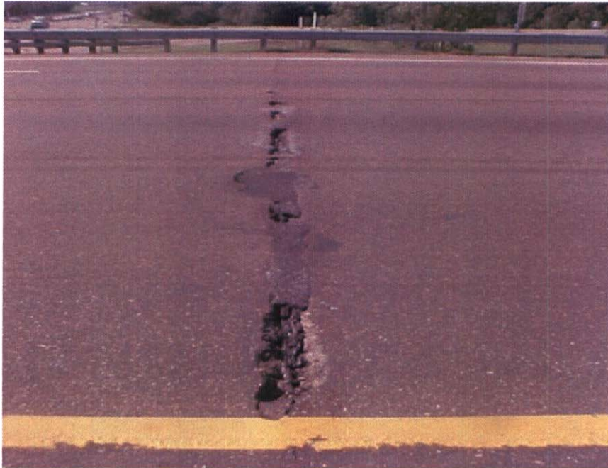
APPROACH #1 PAVEMENT SPALLED
