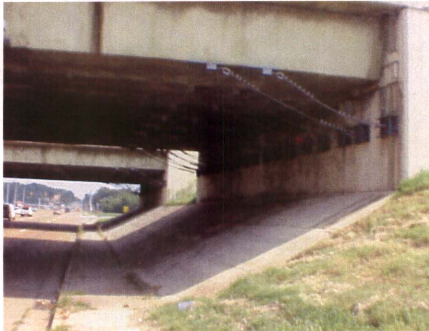
ABUTMENT #2 WITH EARTHQUAKE DEVICE
