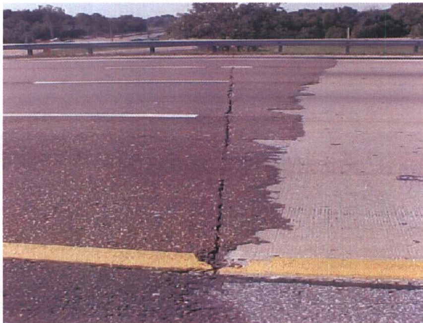
APPROACH #1 JOINT SPALLED
